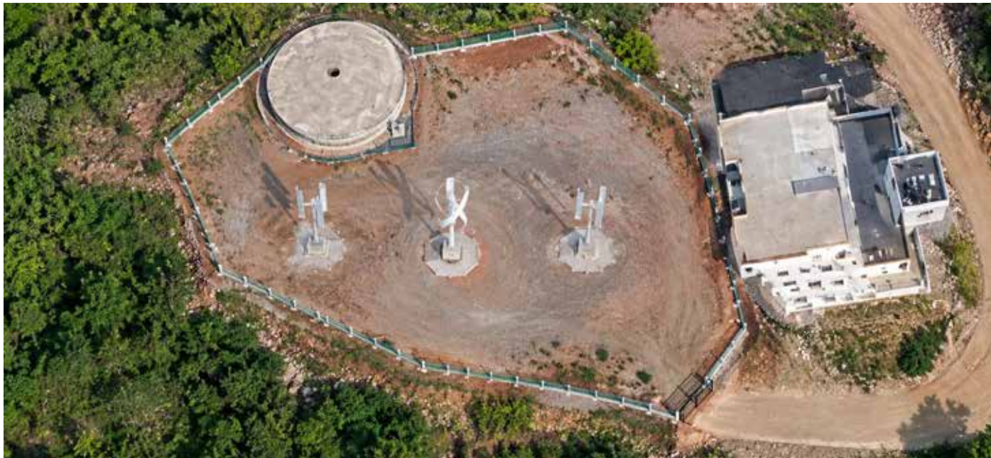
Three vertical-axis turbines on the ridge by the VC Guest House | Drone view, September 2026
