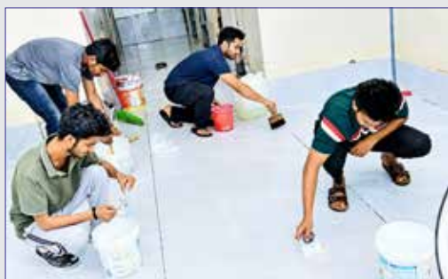
Civil Engineering students at work on the hostel. Photo: Eenadu, 6 Aug. 2026.
